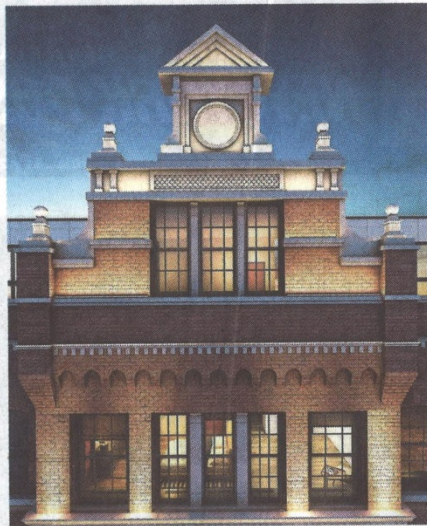
A new light installation at The Schumacher (36 Bleecker St.) spotlights the building's rebuilt pediment crown.
