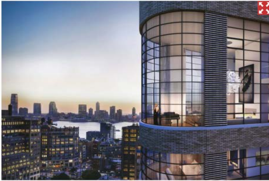
Sleek 10 Sullivan St. is among the showiest of SoHo's new luxury condo developments. Photo: RENDERING
