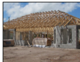
A home in South Florida under construction.
